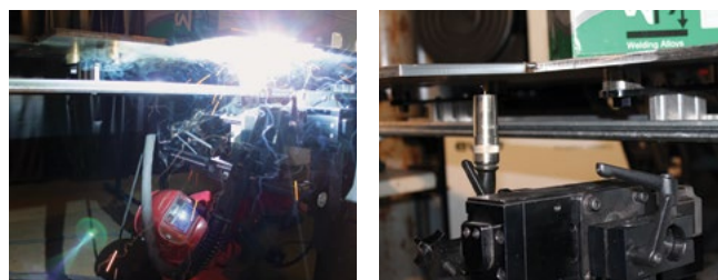
All position welding.
